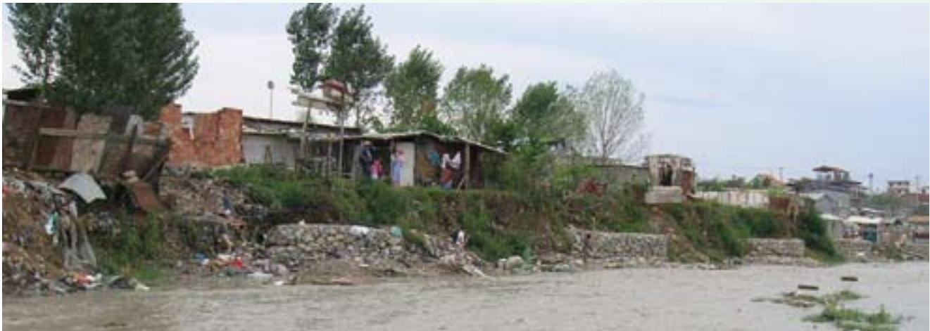
The retaining walls built along the riverbank to prevent flooding of the houses
